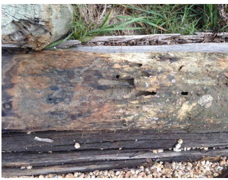
Left: Capped and sleeved pylon. Right Tored worm damage to a timber pylon.
