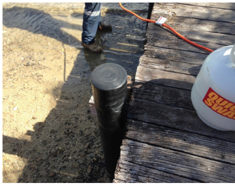
Left: Capped and sleeved pylon. Right Tored worm damage to a timber pylon.
