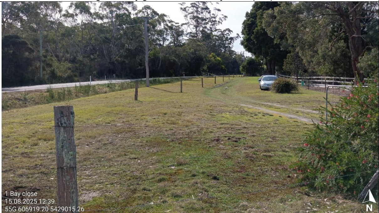
View of existing accessway into the property. To meet the requirements of Table 2, Element B, it needs to be upgraded to all-weather construction.
