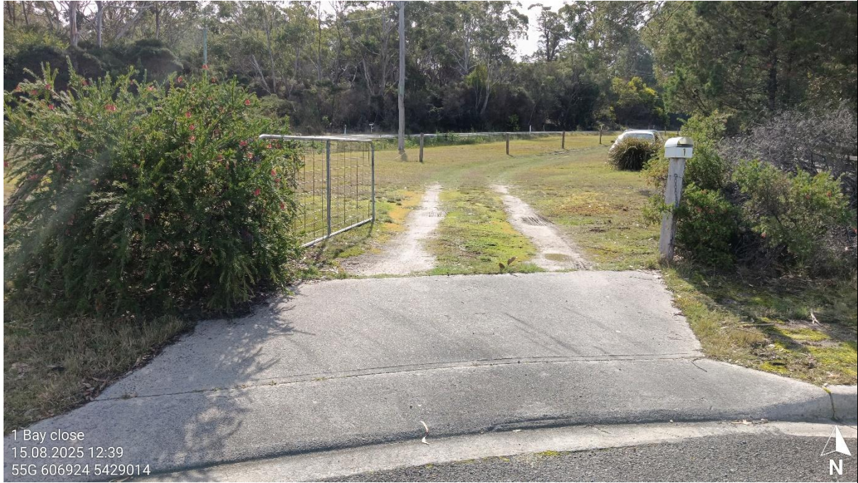
The width of the existing driveway gate at the driveway is 3m (10ft).
