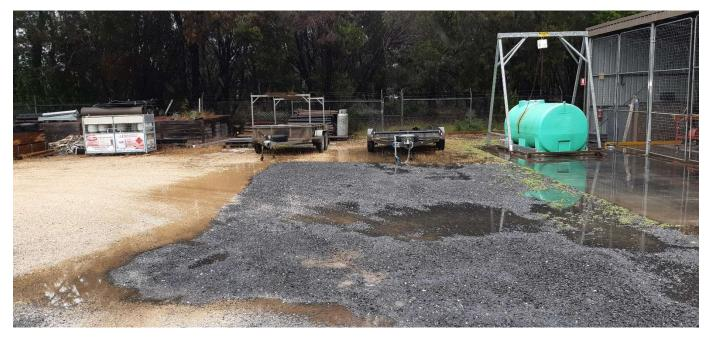
Cate Rear Fence 3m from Vs 1/1 Raised platform vide back fence. Container to be mounted On NEW Perc 400 × 400 × 400 mm concrete Pad s Dangesous on each corner + bolted down. Goods Container New drain Gravelled area. New drain to be dug slauted to # 400 mm Shed Concrete at existing drain, 500mm mide. 7m×12m. pad. Filled with 40 mm clean 3.8m× 12m blue metal. Sump Existing stormwater drain 500 mm wide x 400mm deep. Site Plan - Dangerous Goods Storage St Helens PWS. 1:100 Eagle St, St Helens.
