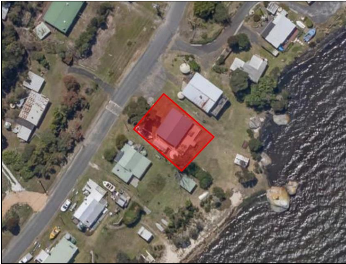
Figure 2: Aerial View of allotment.
