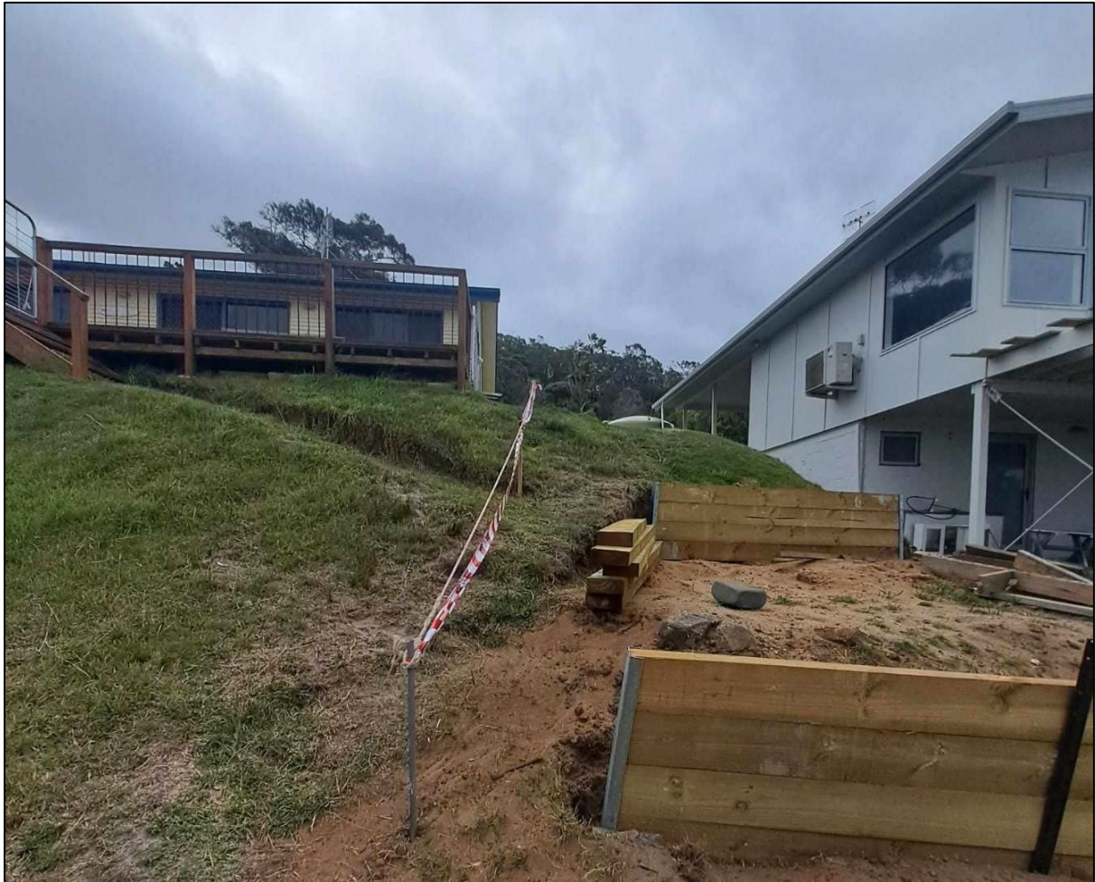
Figure 7: Photo of existing deck (left), illustrating separation between 15 Acacia Drive and 13 Acacia Drive (right).
