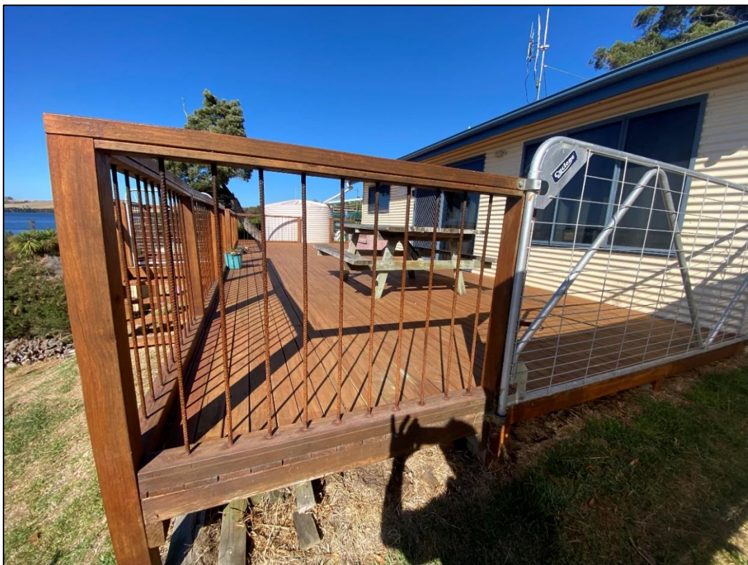
Figure 5: Photo of development site (please note that retrospective works will be completed on the existing deck for compliance with an exemption solution e.g. sub floor enclosure with bushfire screen mesh).
