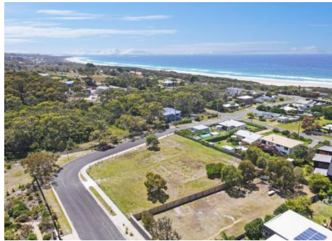
Existing street boundary fence to be replaced:
