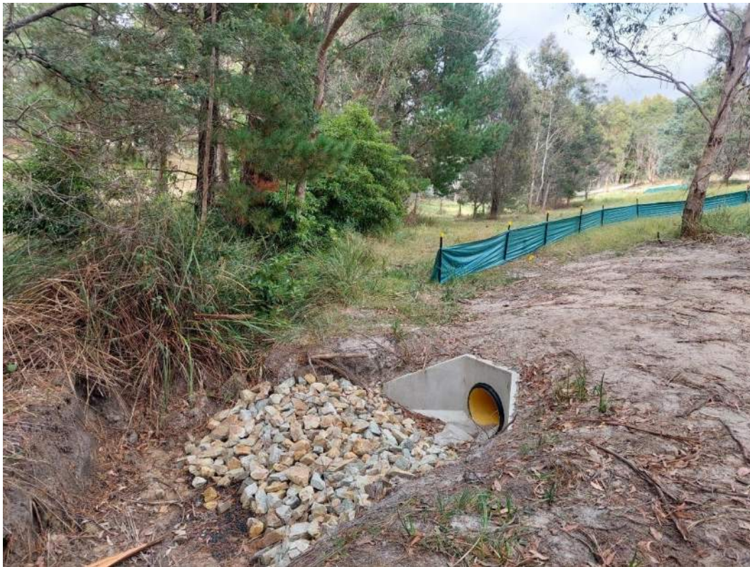
Figure 9: new storm water discharge upstream of development, Council POS
