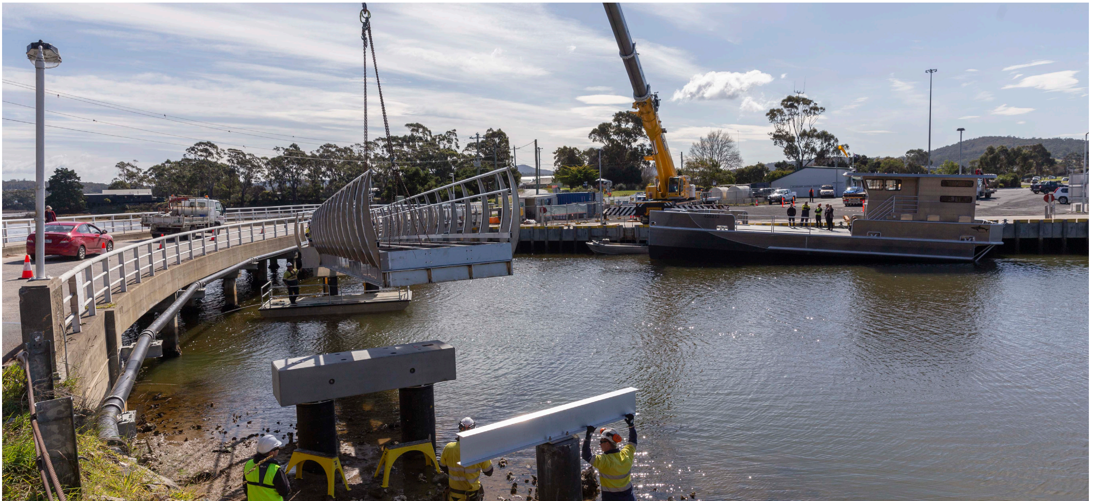
Georges Bay multi-user Track extension - Part of Lyndcraft's custom designed 'whale bone' bridge is lifted into place.
