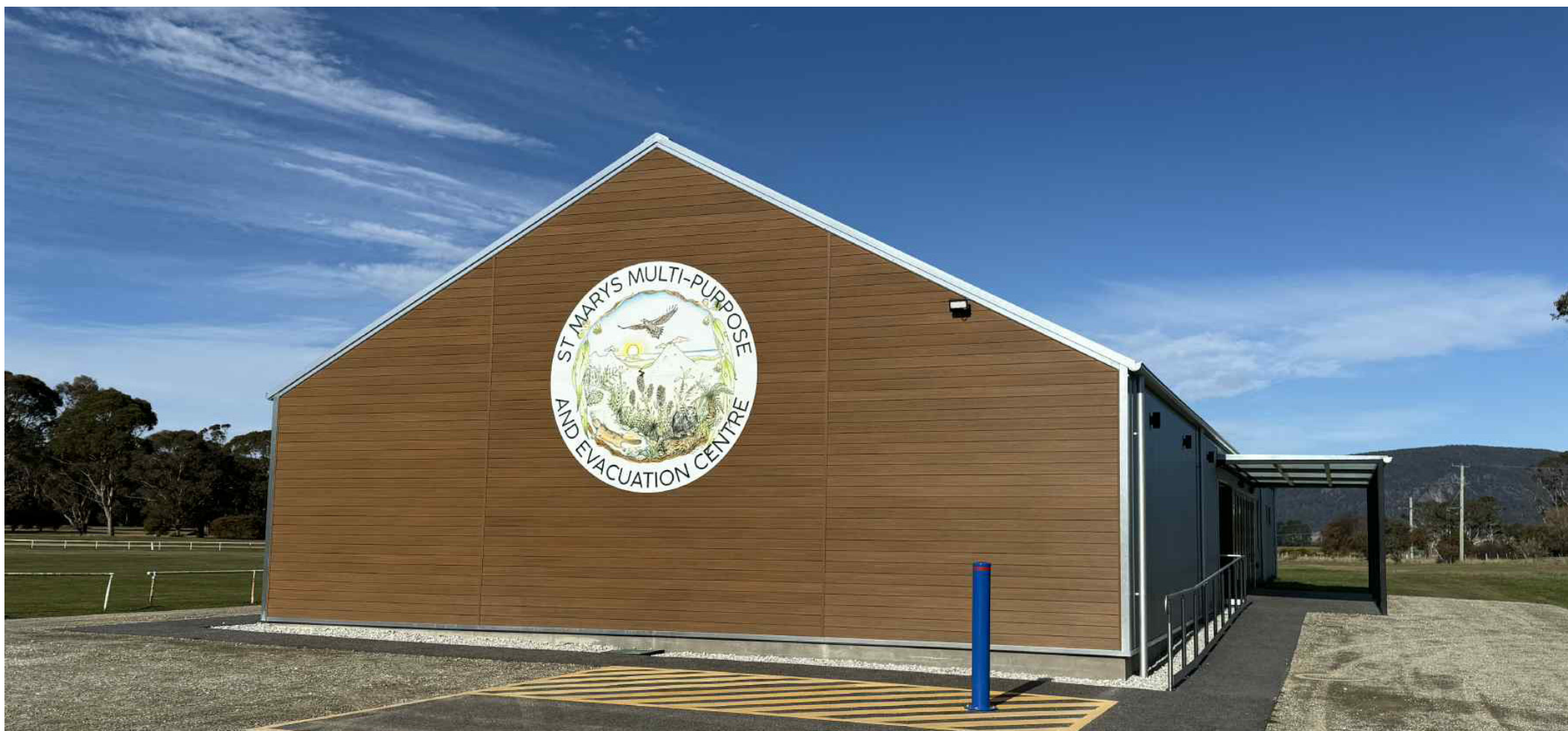
The new St Marys Multi-Purpose and Evacuation Centre with its brand new sign designed by local artist Mel Fidler.
