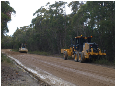
Grading of Ansons Bay Rd has been completed for Easter
