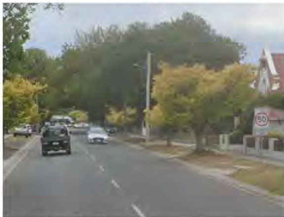
Figure 1 – 50SZ Looking South along Cecilia St approaching CBD
