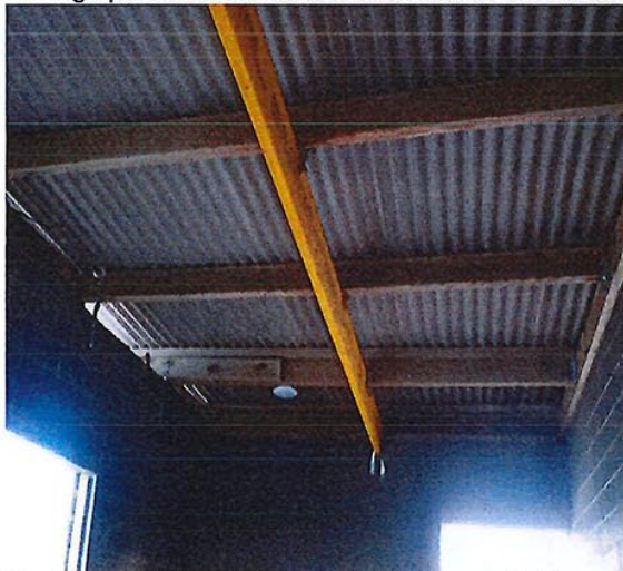
Photograph 10: Roof repair – new tiedowns and rafter
