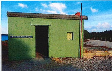
Photograph 6 & 7: North elevation before and after - note lintel and door repairs
