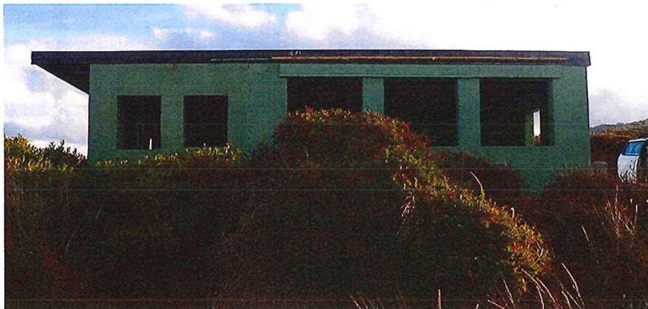
Photograph 2 & 3: East elevation before and after - note concrete lintel repairs and repainting, PWS to request photographs of steel lintels prior to concreting.
