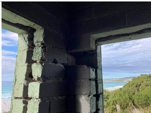
Unsupported wedge of masonry over window (left) Close view of condition of masonry in SE corner (right)
