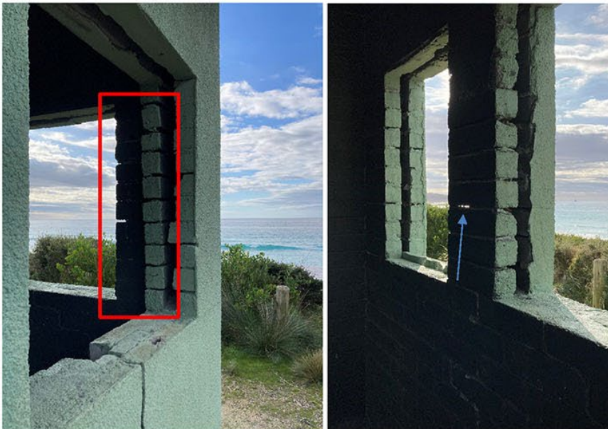
Masonry moving freely (red) unsupported column between windows (blue)
