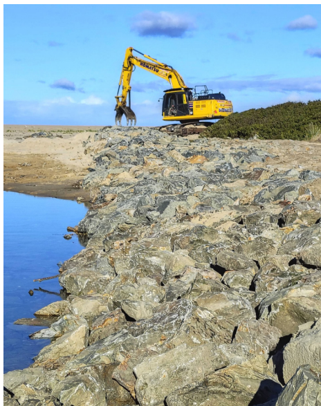
Photo: Rock wall being repaired at the River Mouth
