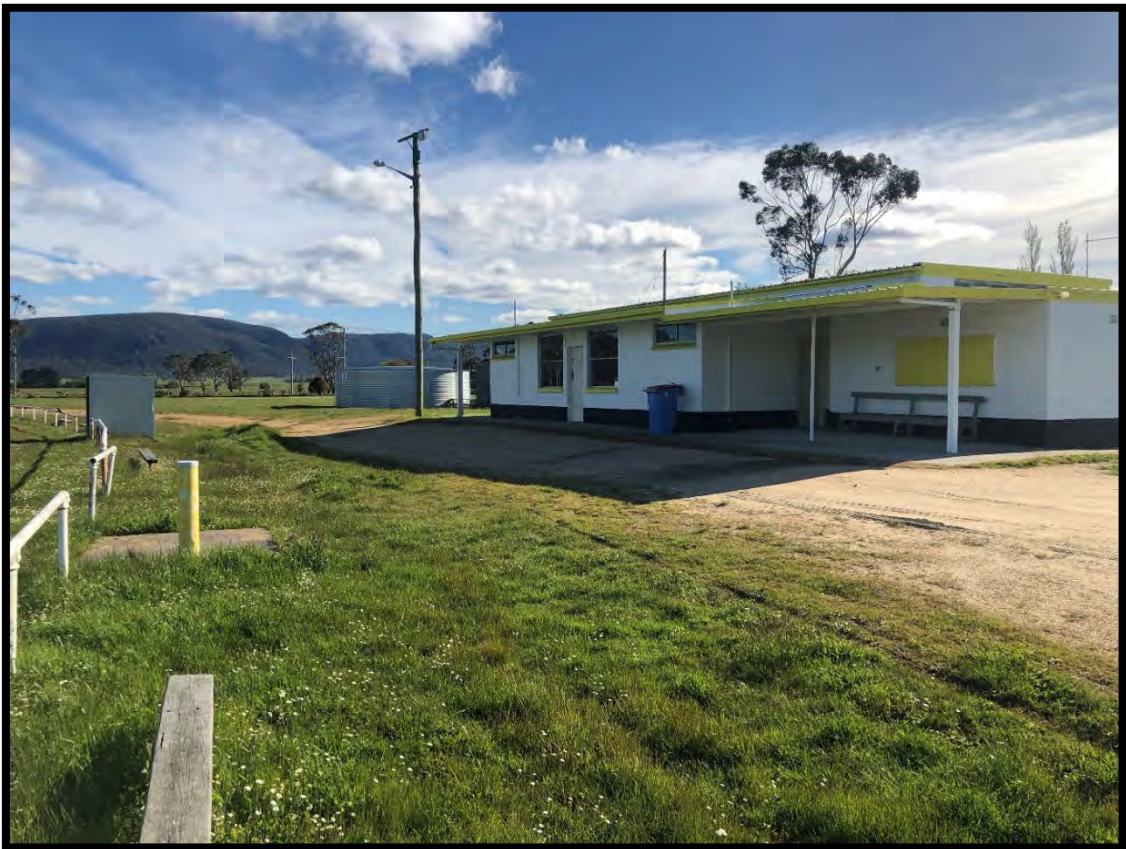
^Area east of building looking toward Reservoir
