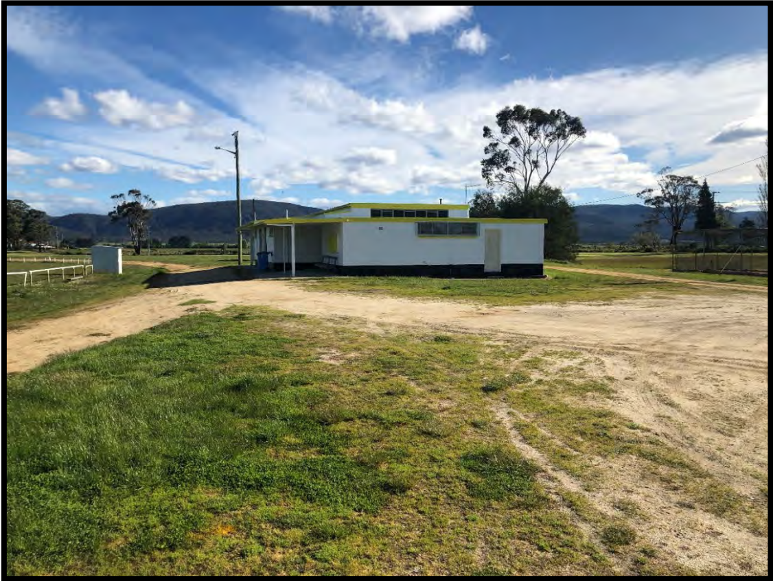
^Existing Structure to be demolished
