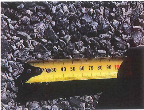
Figure 3.6 – North Ansons Bay Rd seal condition near Accacia Drive
