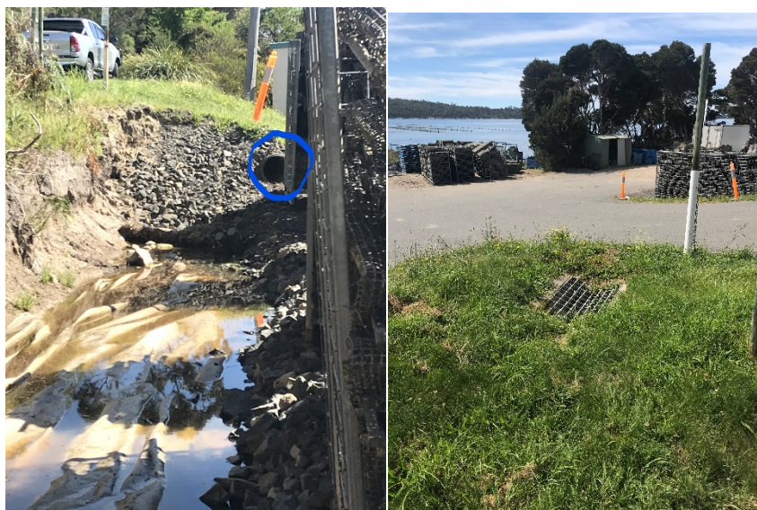
Figures 6 & 7 Stormwater Pipe to be reconnected - drainage from road reserve
