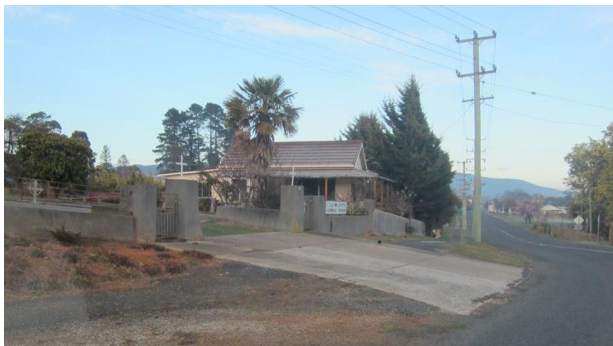
Figure 14 (top left): Changing Footpath Grades due to Driveway
