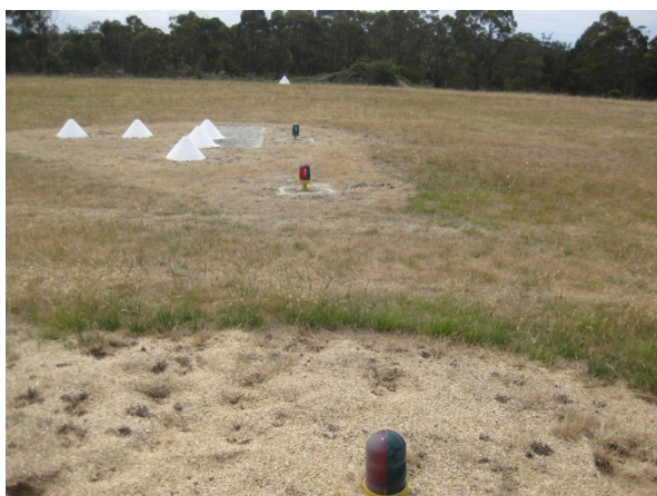
Photo 7 – Existing Runway Threshold Lights
