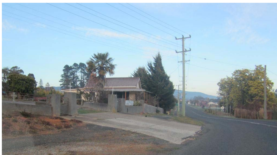
Figure 3.17: Changing Footpath Grades due to Driveway
