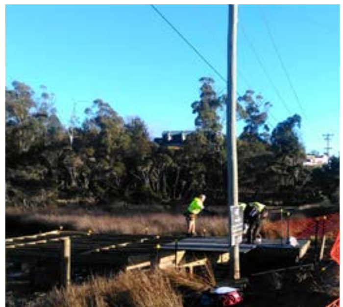
Construction of the Boggy Creek Board walk is well underway
