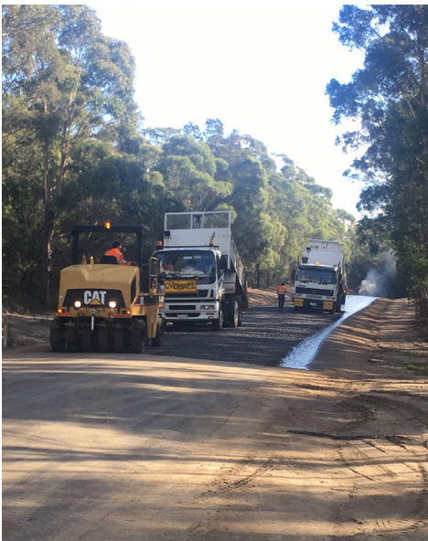
The works Team undertaking Road Sealing.
