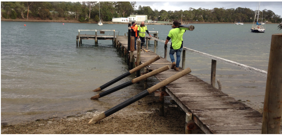
Council workers at the Talbot St jetty replacing pylons.
