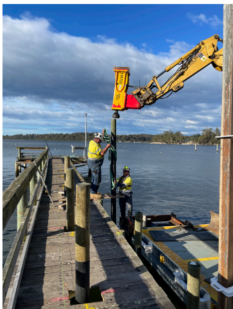
Pictured Below - Pile driving at Kirwans Jetty
