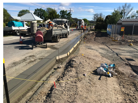
Kerb and Channel installation in Annie St, St Helens.
