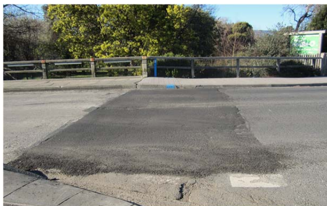
Figure 19: Bridge Condition in St Marys
