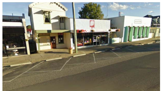
Figure 32: Kerbing Too High
