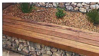
GABIAN STONE BASKET: SEATING OR LOW WALLS, TIMBER TOP SEATING
