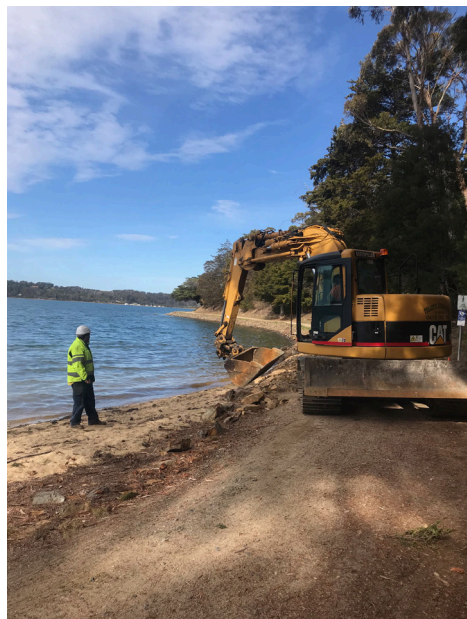
Works crews reinforcing the rock wall around the Georges Bay multi-user track.
