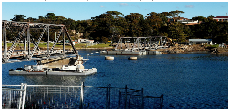
The Old Scamander Bridge with the middle section removed. Image courtesy of George Keri
