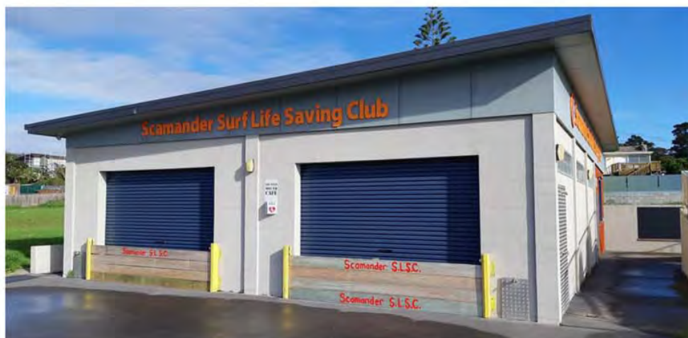
FIGURE 37: POST AND PANEL BOARDS AT SCAMANDER SLSC
