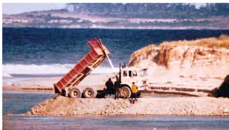
FIGURE 33: CONSTRUCTION OF THE TRAINING WALL IN 1989
