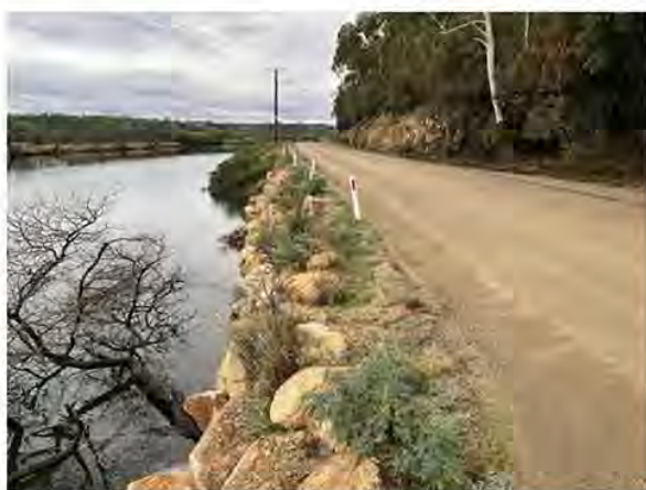
FIGURE 31: RIVERBANK ROCK PROTECTION ALONG UPPER SCAMANDER ROAD (PHOTO BY N. LEWIS)
