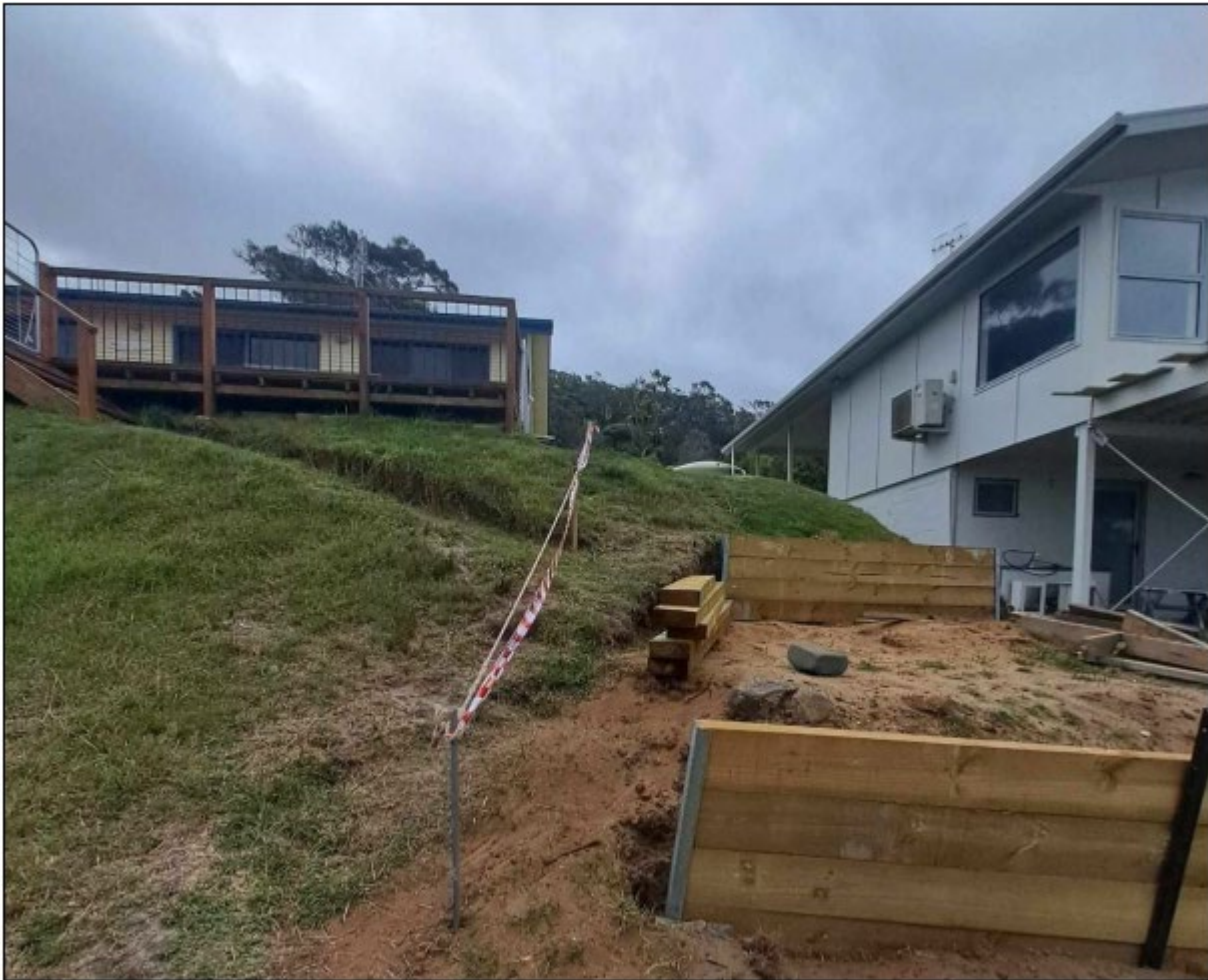
Planning Ahead Tasmania, Existing Deck – Supporting Submission, Figure 7: Photo of existing deck (left), illustrating separation between 15 Acacia Drive and 13 Acacia Drive (right).
