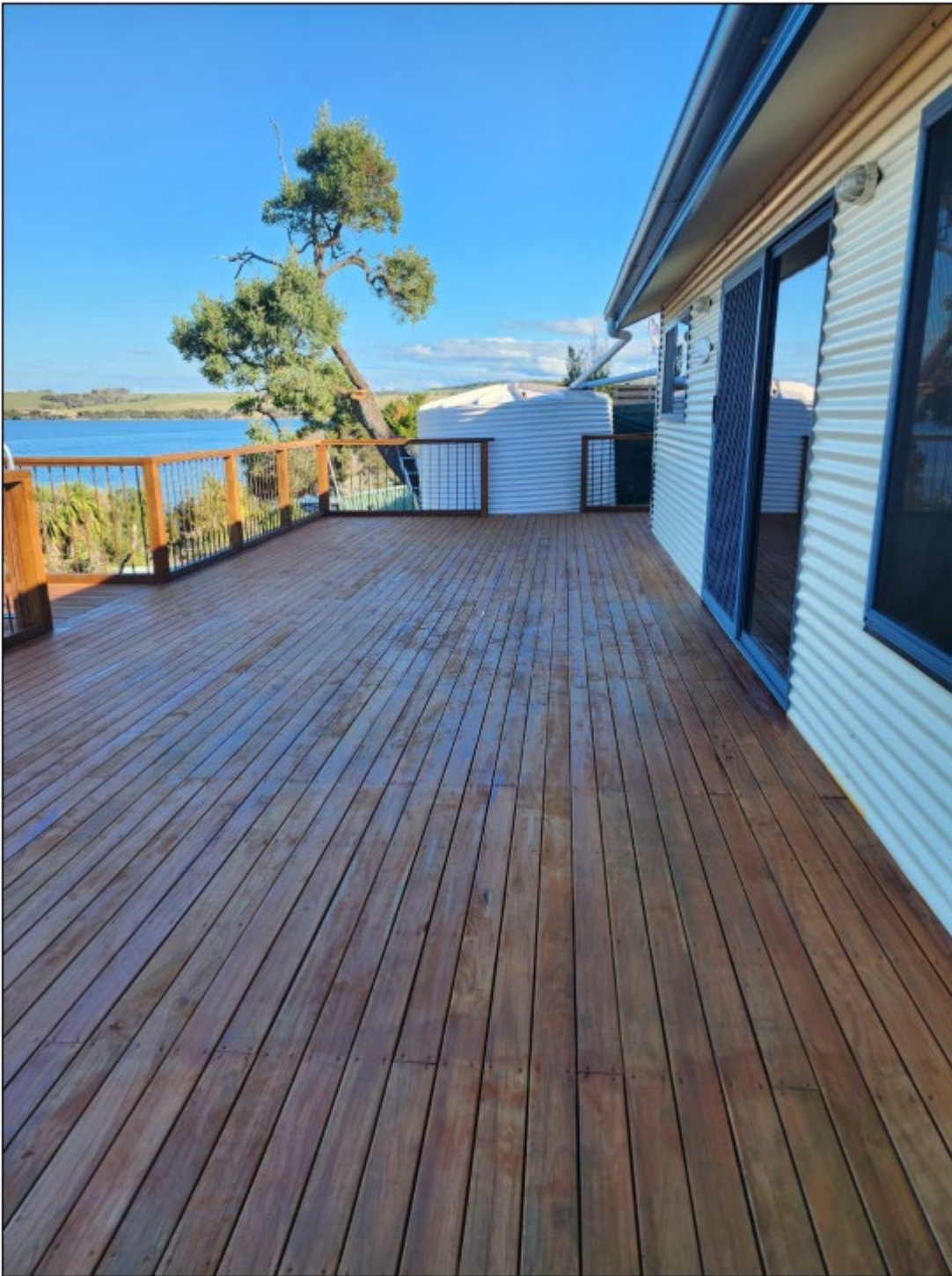
Planning Ahead Tasmania, Existing Deck – Supporting Submission, Figure 6: Photo of deck looking southwest (photo taken May 2025)
