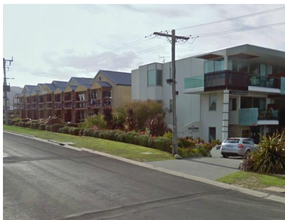
PICTURE 2 – 2-3 STOREY HOLIDAY ACCOMMODATION, APOLLO BAY
