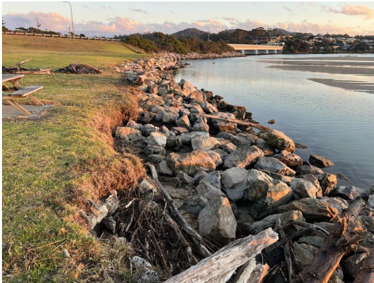
FIGURE 35: FORESHORE EROSION PROTECTION ROCK WALL (PHOTO BY N. LEWIS)
