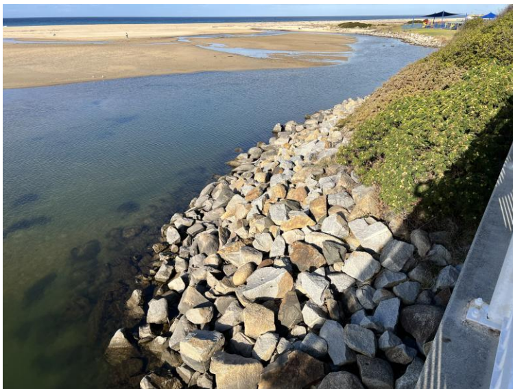
FIGURE 34: BRIDGE ABUTMENT SCOUR PROTECTION (PHOTO BY N. LEWIS)
