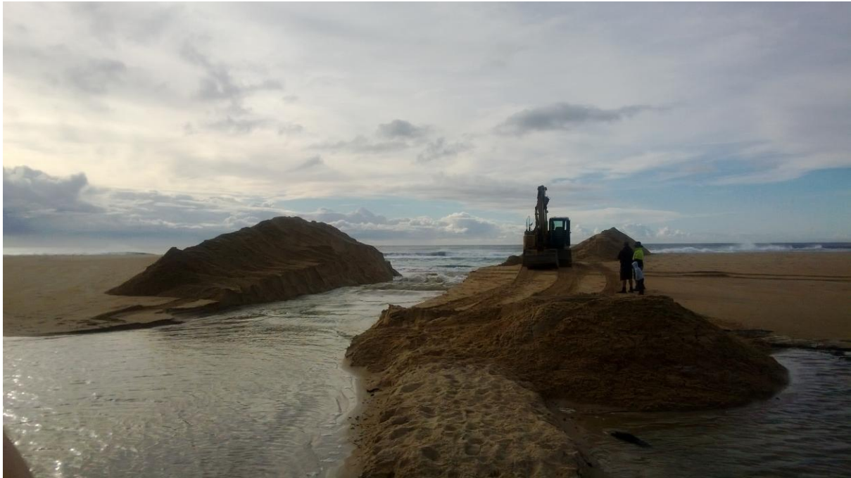
FIGURE 36: BARWAY OPENING PROCEDURE (AT COMPLETION)
