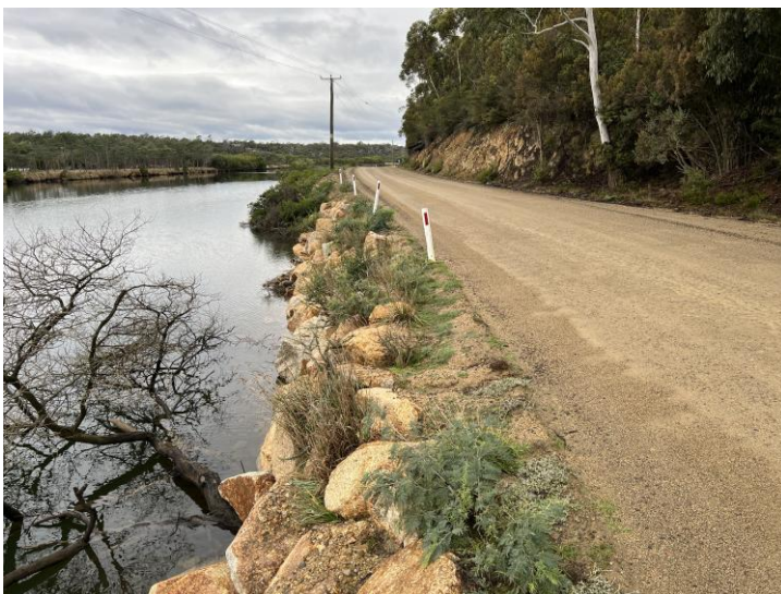
FIGURE 31: RIVERBANK ROCK PROTECTION ALONG UPPER SCAMANDER ROAD (PHOTO BY N. LEWIS)
