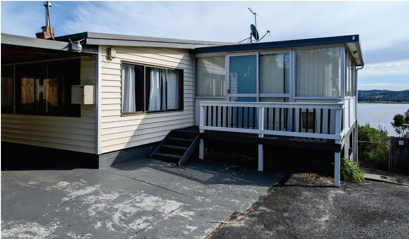
Plate 4 - View of the existing dwelling looking to the east
