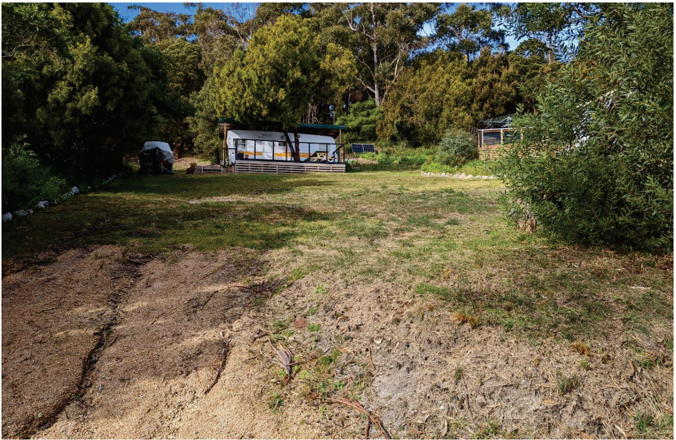
Plate 3 - Shallower slopes within affected area of the landslide ID 5080, immediately to the northwest of the site
