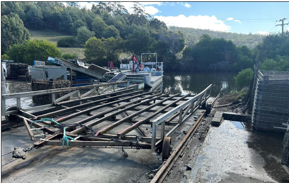
Figure 6: Image of existing slipway servicing site, to west (approx. 15 metres) of proposed slipway footprint (photo taken 31/07/25).
