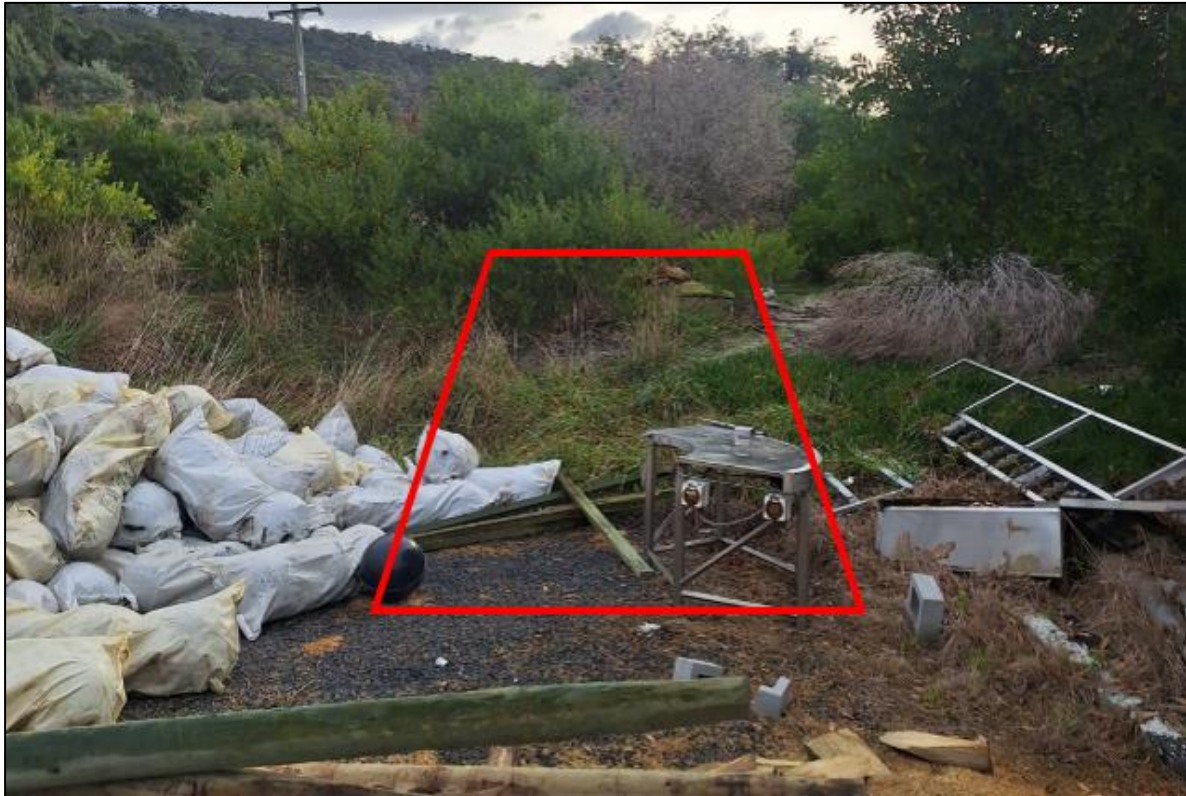
Figure 5: Image detailing site and approximate footprint location of slipway (photo taken 23/07/25).
