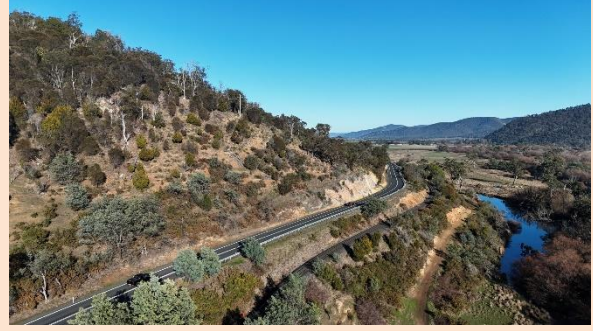
Aerial imagery – Lot 1 looking to west
