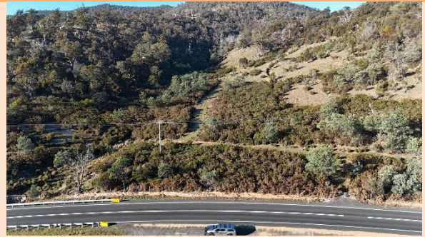
Aerial imagery – Lot 1 looking to south
