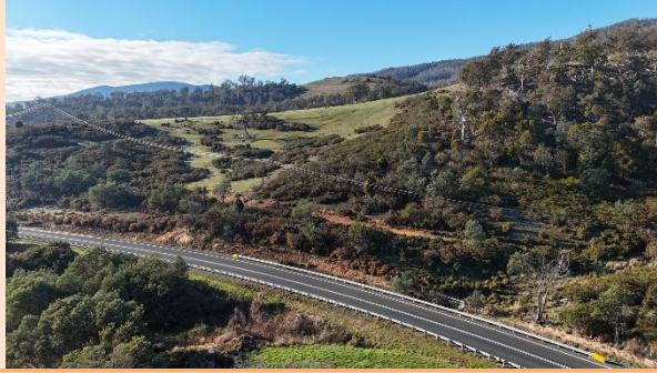
Aerial imagery – Lot 1 looking to southeast
