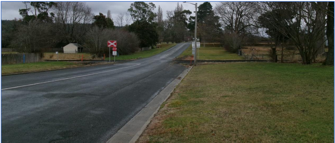
Photograph 8.3B – Available sight distance to the right of the new access
