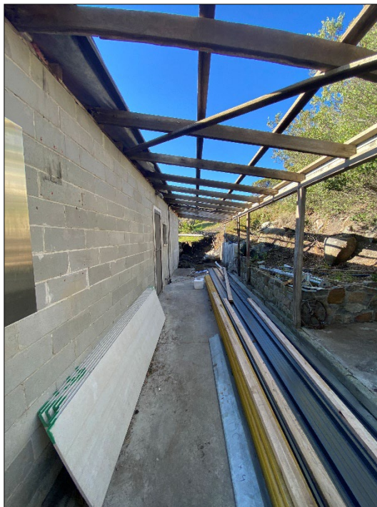
Photo 2 Rear existing attached verandah
