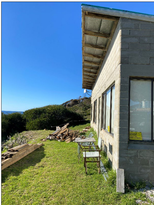
Photo 1 North facing existing dwelling
